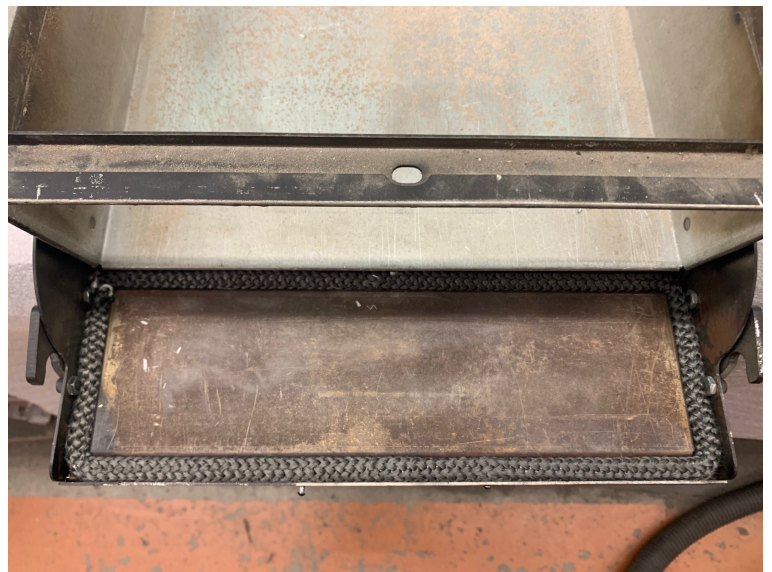
New gasket applied and ends joined to eliminate any gap
