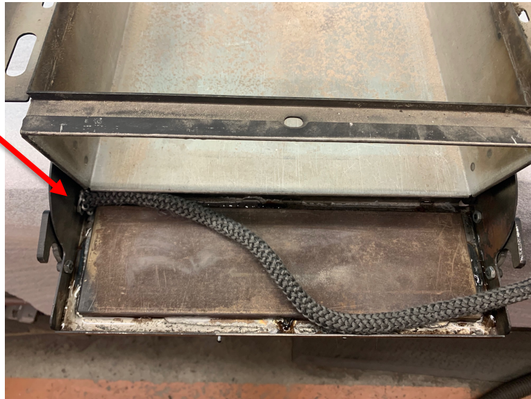
Install the new gasket starting at one of the corners closest to the stove
